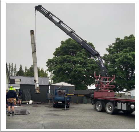
Old chimney making way for our new boiler instalment.
